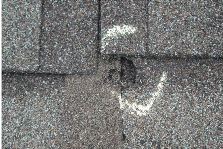
Figure: Hailstorm damage on a roof. Source Rapid Roofing 2024 ( https://rapidroofing.com/blog/identifying-and-repairing-hail-damage-to-roof-a-homeowners-guide/ ).
