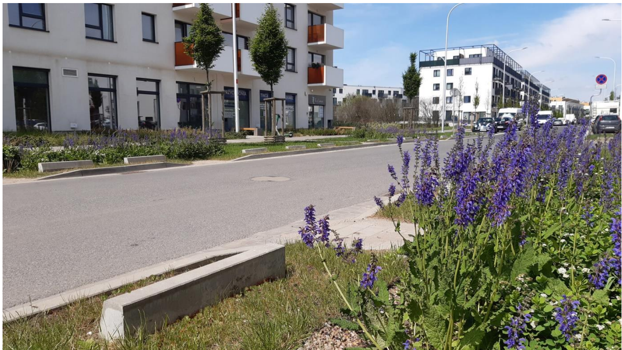
Fig. 3 Local stormwater management in a rain garden collecting runoff from S. Drabika Street, Wrocław (Poland). (Photo: J. Rubaszek).
