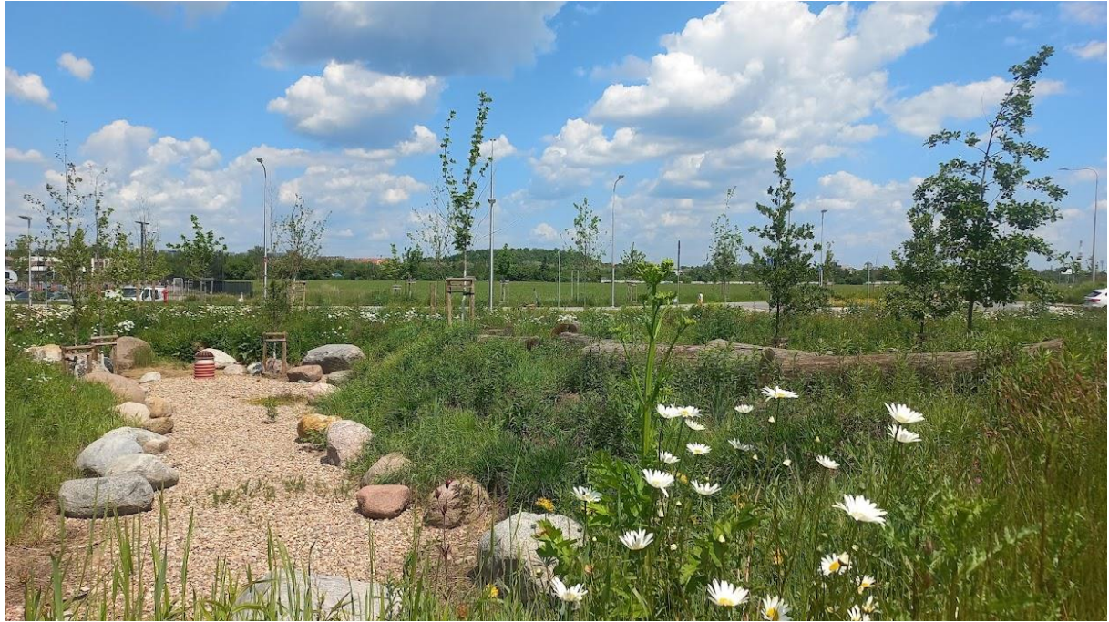
Fig. 2 Infiltration swale on Asfaltowa Street in Wrocław (Poland), designed to collect excess water during heavy rainfall (Photo: J. Rubaszek).
